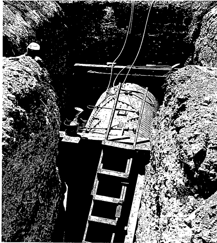
Fig. 3—Exterior views of pipe in place before placing backfill.
